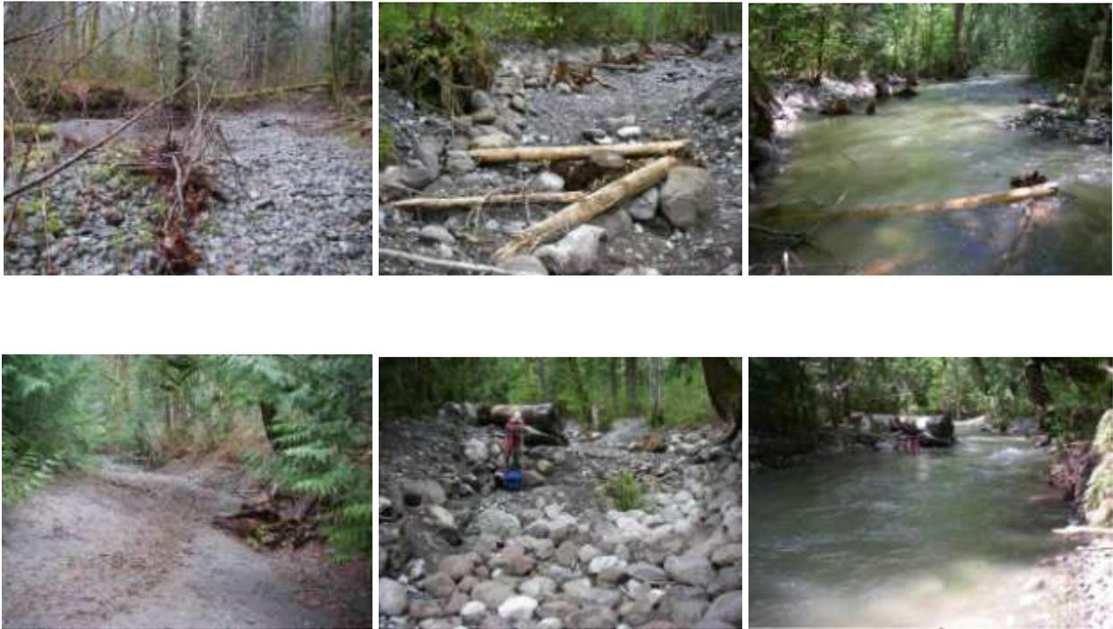
Figure 3.17.—Photos of the Cheakamus River km8 Side Channel Rewatering Project showing pre-construction, during construction and nominal flow conditions ( $90 \text{ m}^3/\text{s}$ ) after construction. Physical habitat elements such as boulders and large woody debris were important features incorporated into the design.
